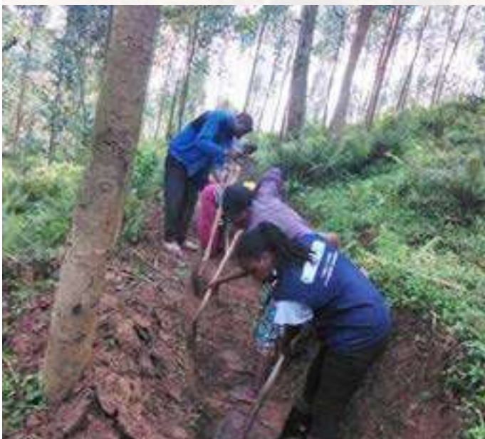
The maintenance of trenches belongs to beneficiaries (Photo: Liliane)
