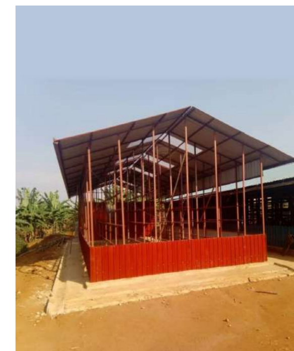
New Hangar constructed by KODUIBI in 2019
