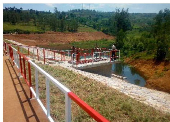
Bridges constructed in sectors of Muganza and Mugombwa for crossing the Musizi marshland.
